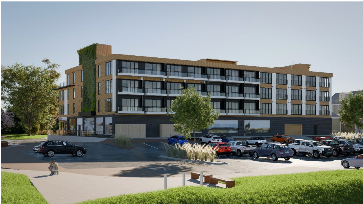
Image 4: 292 Main Street – looking South from the Rail Line at the rear of the building/parking lot.
