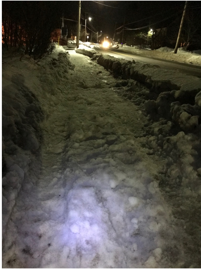
IMG8875 - Feb 11, 9.27pm - 7 days after freezing rain/ice storm?
