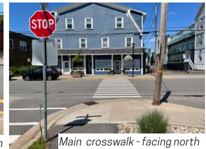
Main crosswalk - facing north
