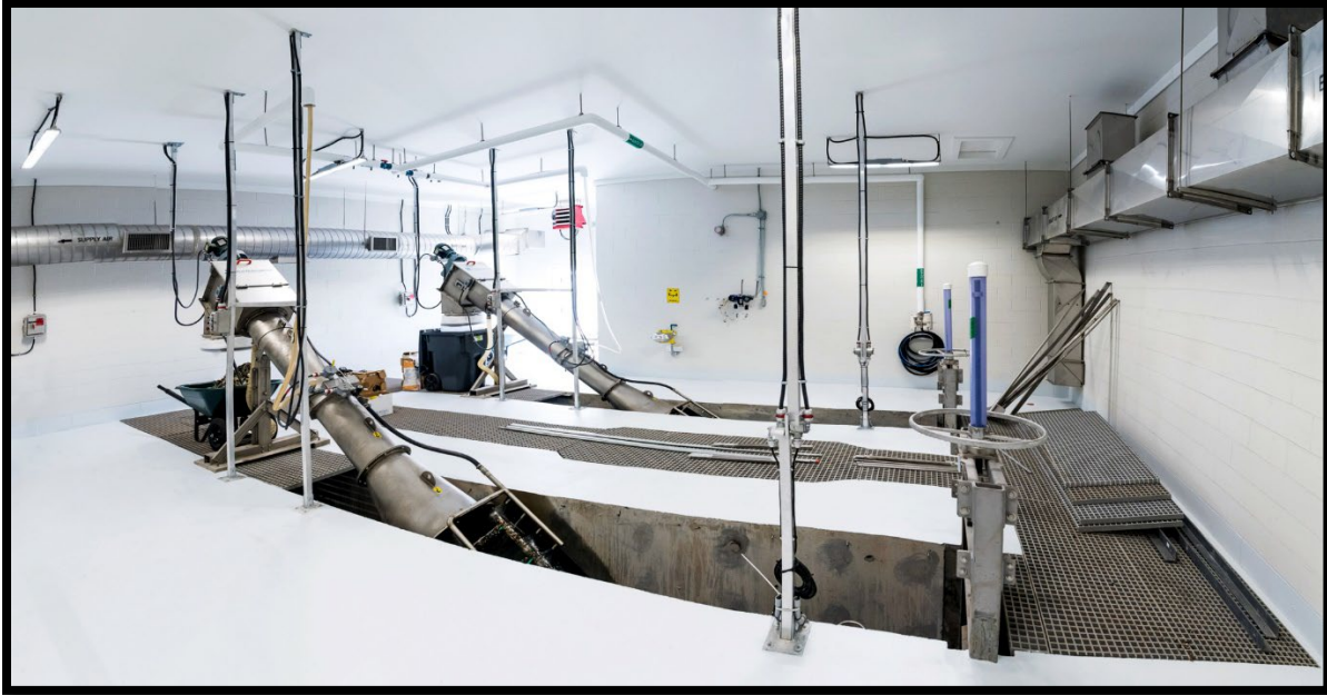
Figure 2-1. New Screening Building
