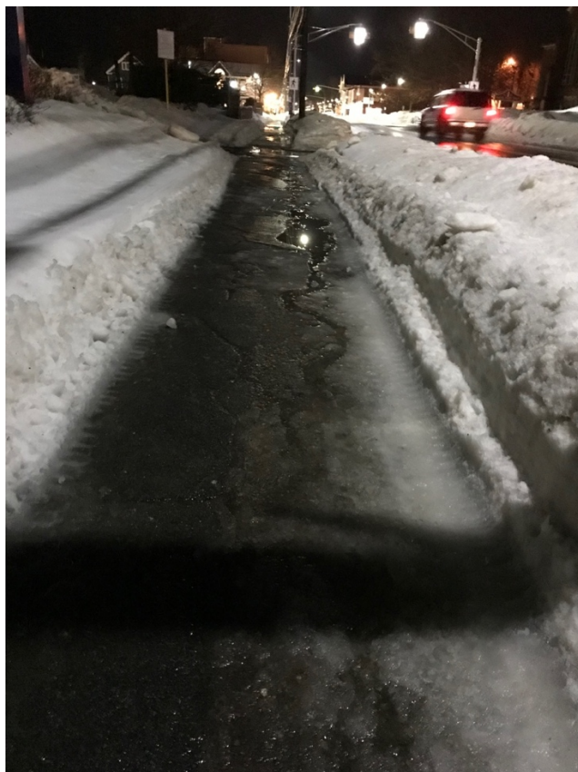
IMG8405 - Feb 8, 9.06pm – snowbank trapping water which then freezes, icy need to add traction
