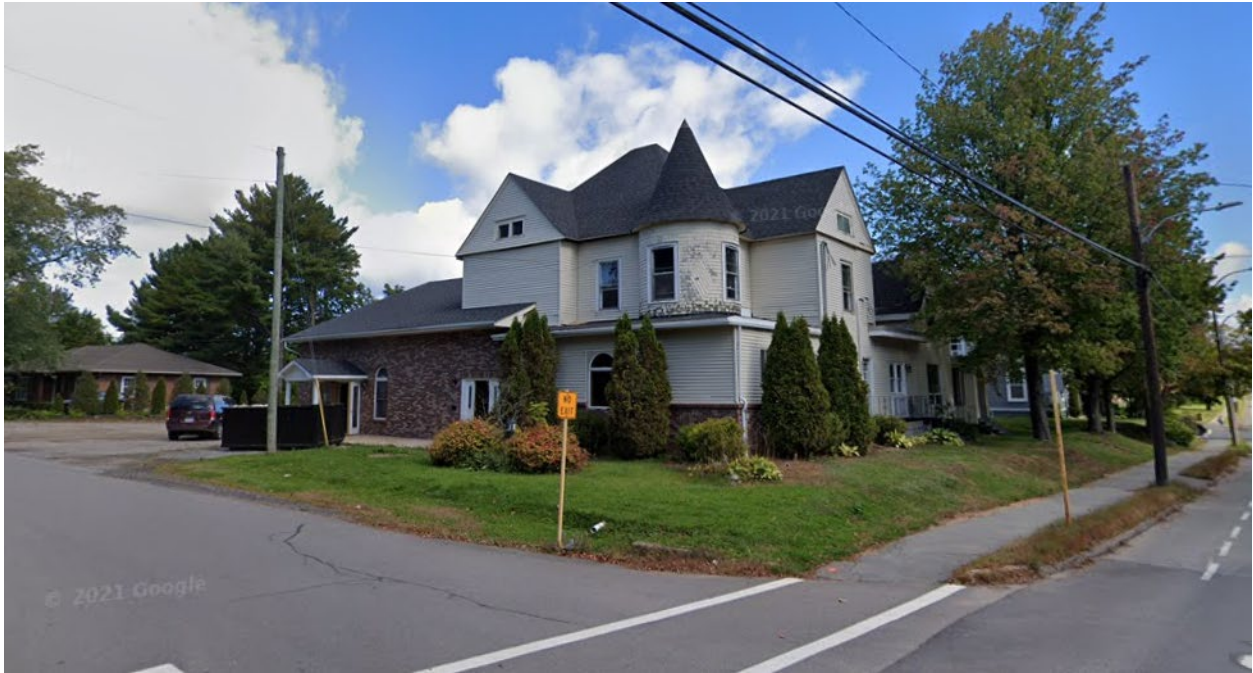
Figure 4: 568 Main Street - Main Street View looking east
