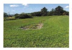
The existing detention pond (photo) in the Northwest the corner of Viking development is designed, and has demonstrated that it is capable of retaining peak storm water flows for the south eastern portion of the development.
