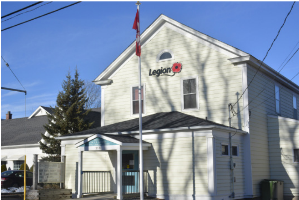
The exterior of the Legion building, after renovation
