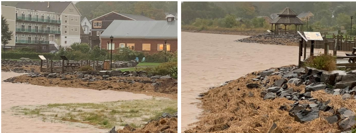
Figure 7.1: Photos of High Coastal Water Levels During Hurricane Teddy
