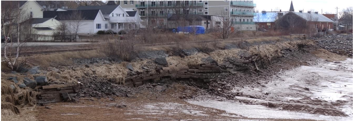
Figure 8.3: Erosion on the Bank by the Railroad
