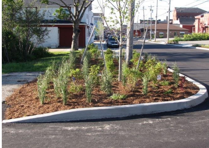
Figure 40: Vegetative Filter Strip Example
