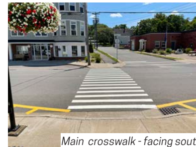
Main crosswalk - facing south
