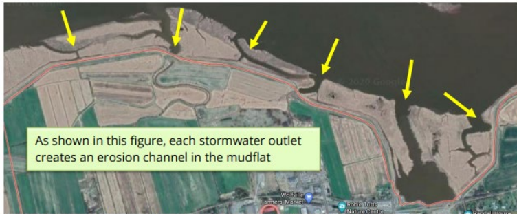
Figure 8.4: Typical Erosion Patterns in the Mudflats Originating at Stormwater Outfalls
