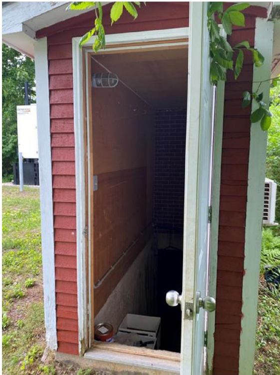
Figure 3- Existing East Side Basement Door
