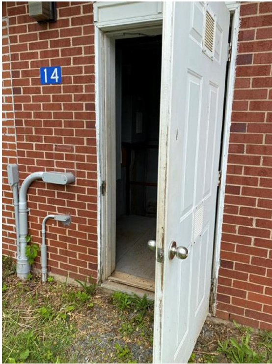
Figure 2 – Existing South Side door
