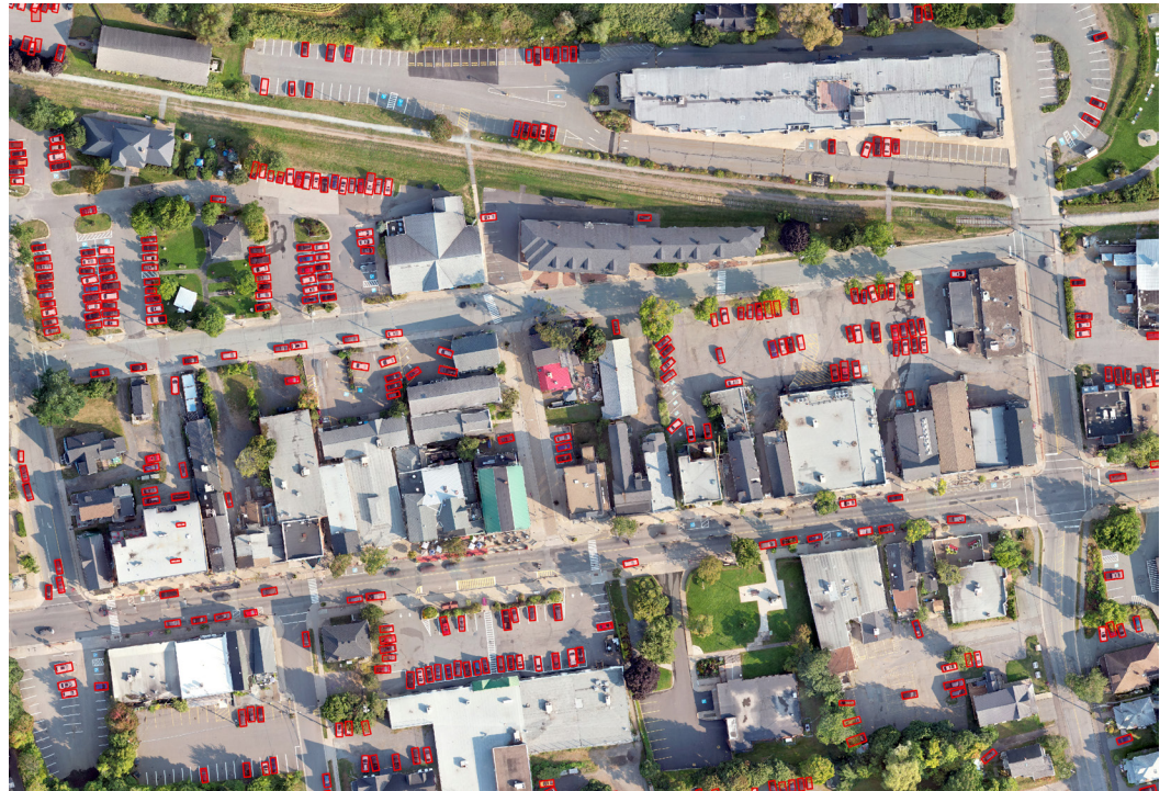
Figure 5 — Core Concept for New Town Owned and Operated Parking (Implementation Framework), this also supports policy direction in the Investment for Success section of this MPS (Part 3)
